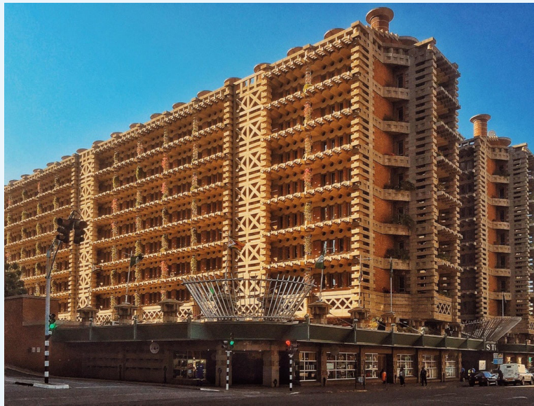
Living Spaces: Watch how the Eastgate Center in Zimbabwe Cools Itself Without Air Conditioning
